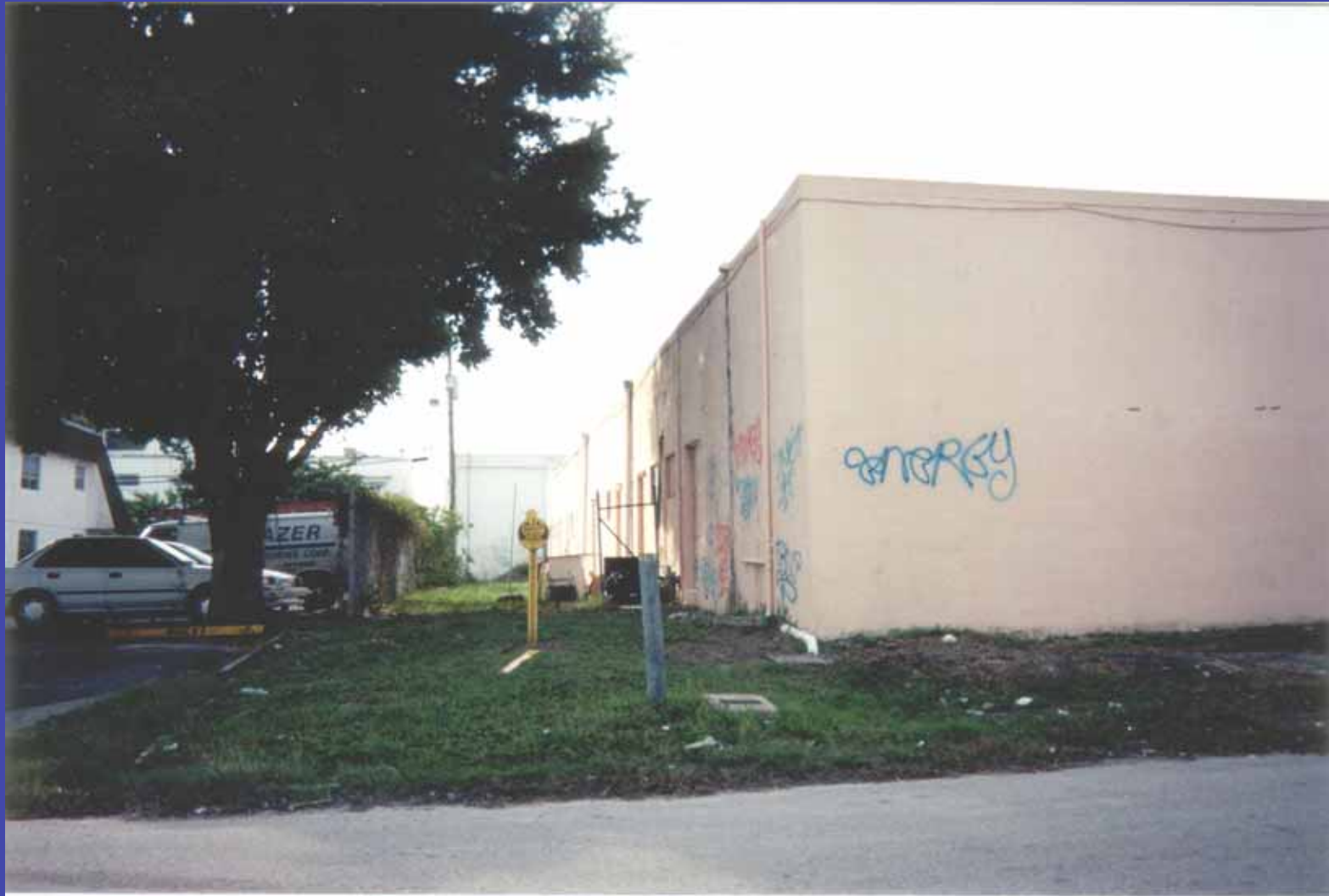
Everglades Pipeline - Business at U.S. 441 Crossing (Looking South)
