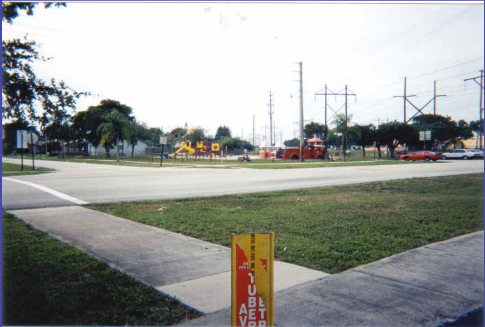
Everglades Pipeline - Pipeline Through Playground at Johnson Street (Looking SW)
