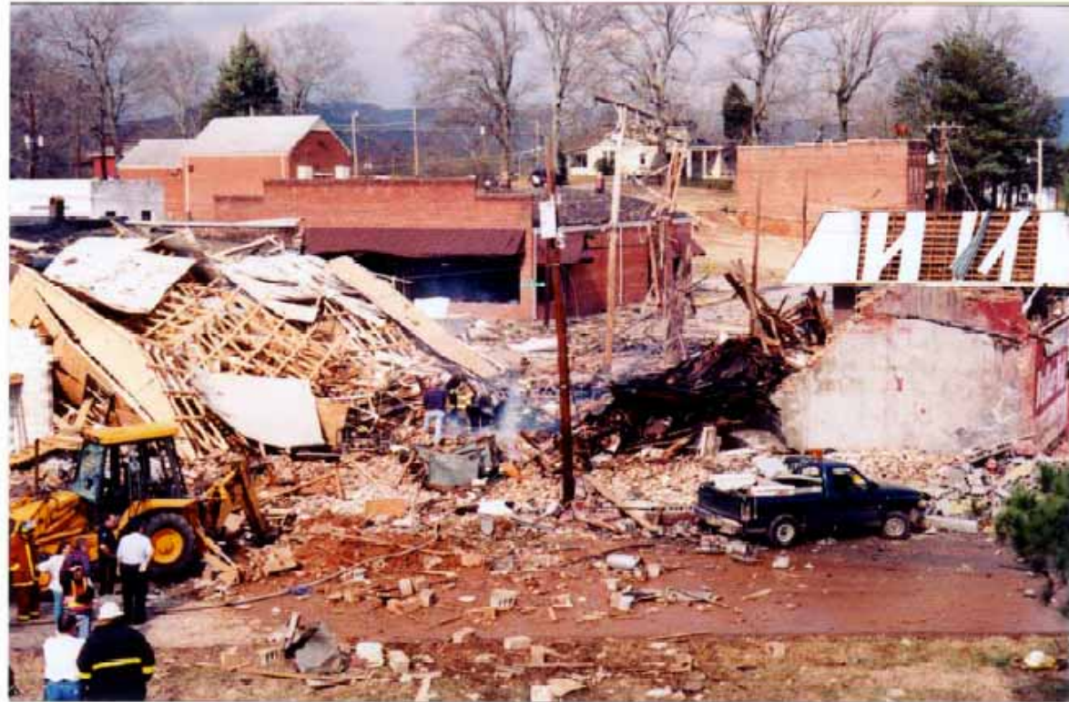
Figure 2. Damage to 404, 406, and 408 Alabama Avenue
